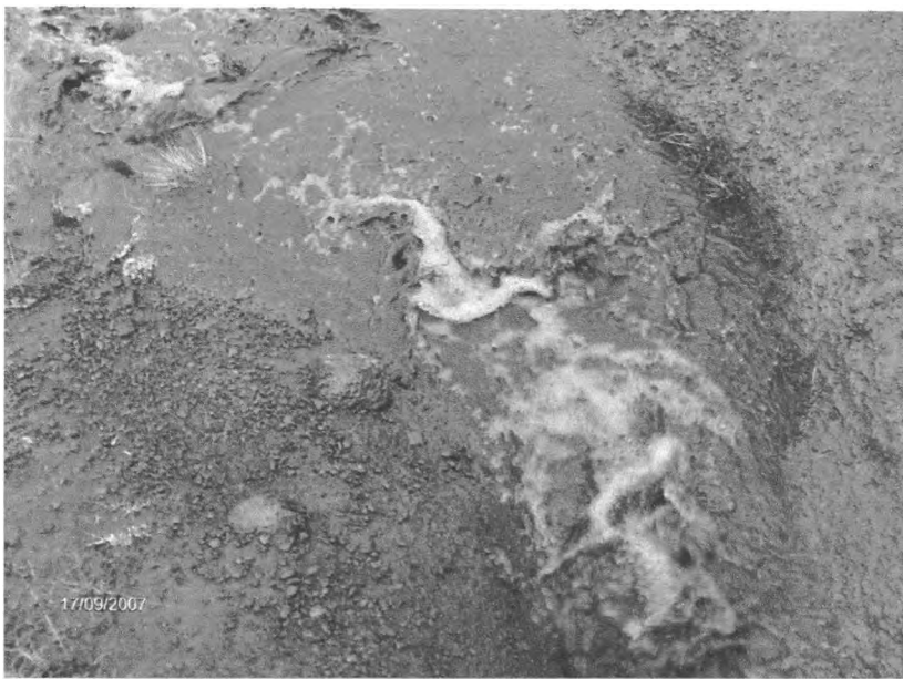
Figure 4: Gully erosion on Old Moses-Likii North trail
