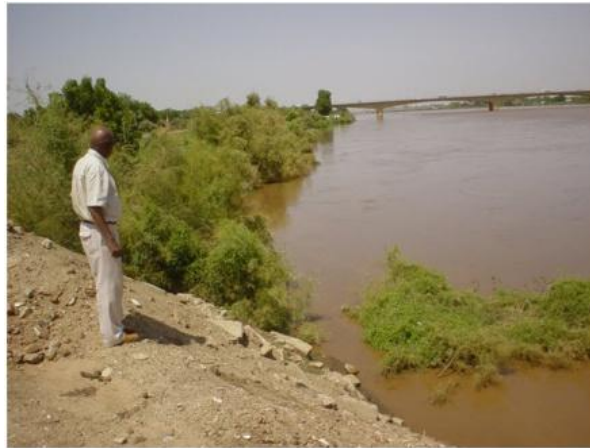
Figure 5-5: Blue Nile eroded bank
