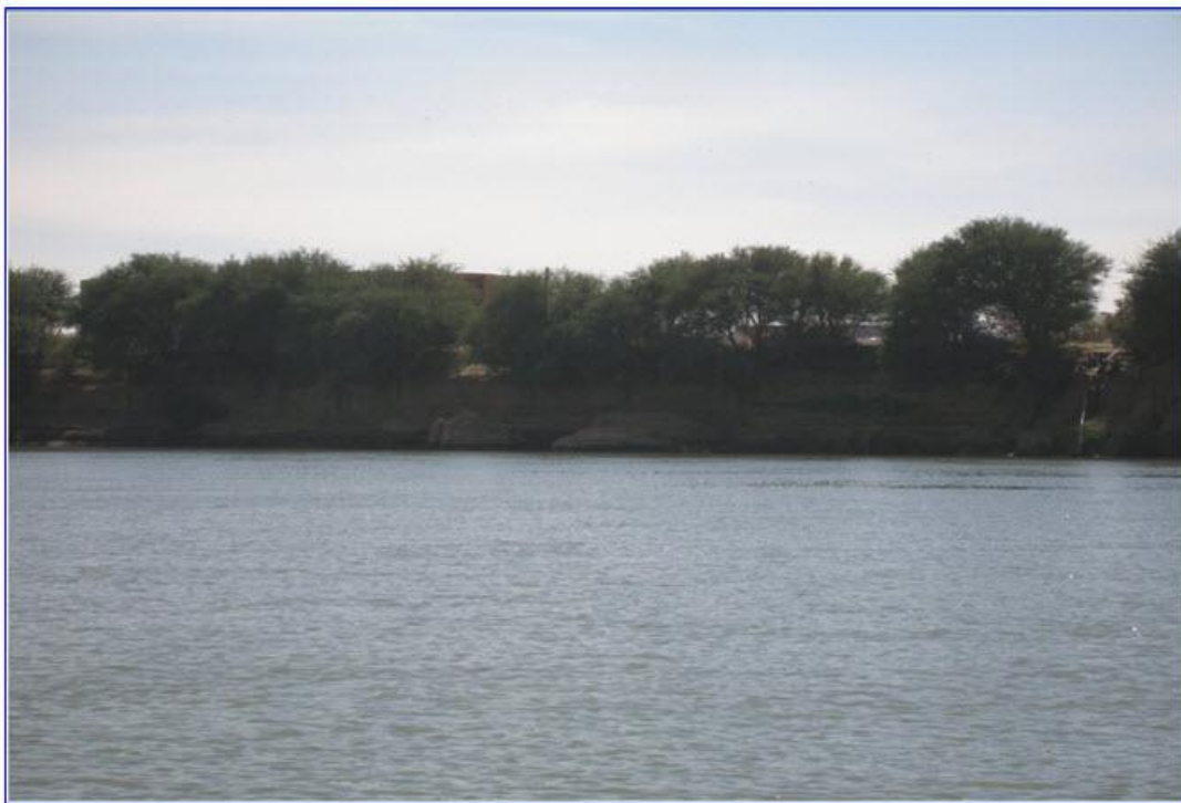
Figure 6-11: Erosion of the western bank upstream of bridge site
