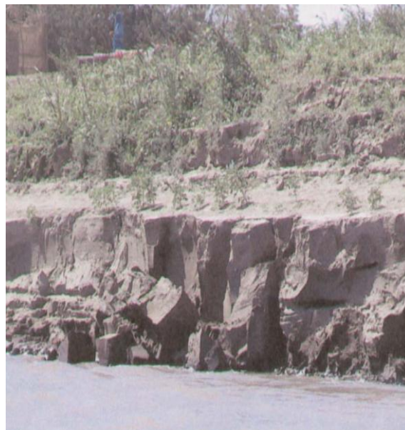
Figure 3-6 : Bank erosion – failure as a beam type in Northern State (Karima – Dongla Reach)
