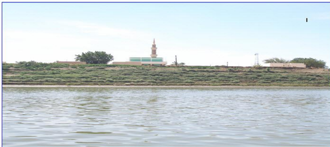
Figure 6-9: Western Bank D/S of the Proposed Bridge
