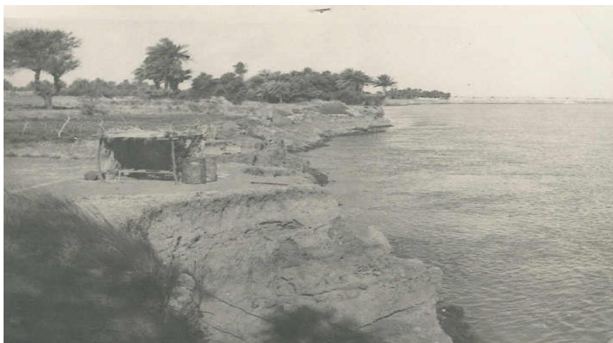
Figure 2- 2: Very Severe Bank Erosion Dongla – Merowi Third Reach
