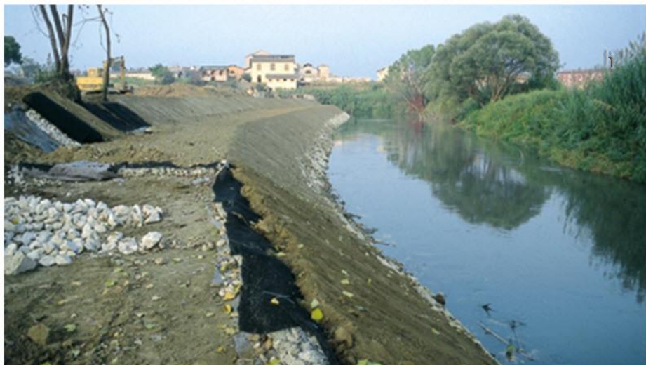
Figure 5-15: Typical gabion groynes in construction
