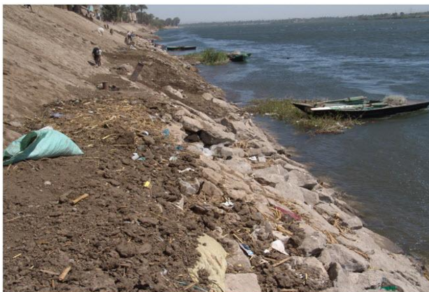
Figure 6-2: General view of bank toe protection
