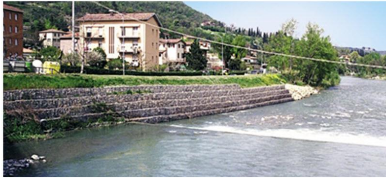
Figure 5-14: Typical guide bank gabion walls
