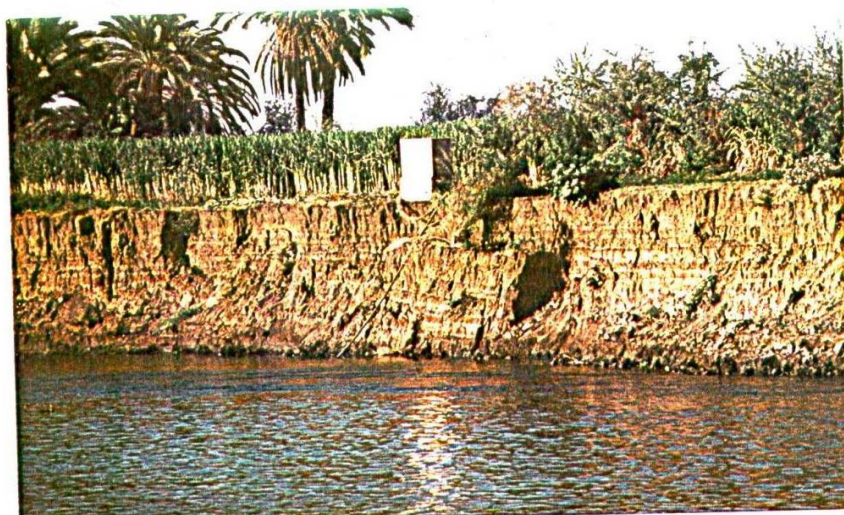
Figure 2- 1: Typical Bank Erosion at Luxor
