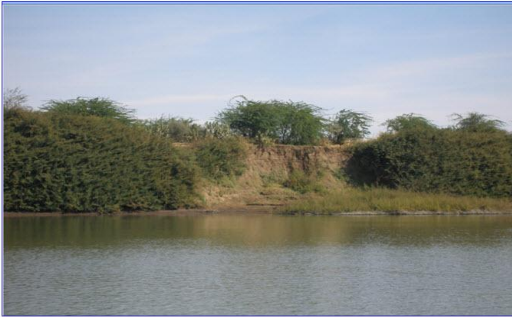
Figure 6-10: Erosion of the eastern bank upstream of the bridge site
