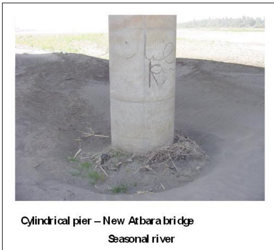
Figure 6-17: Live bed scour in the Nile River
