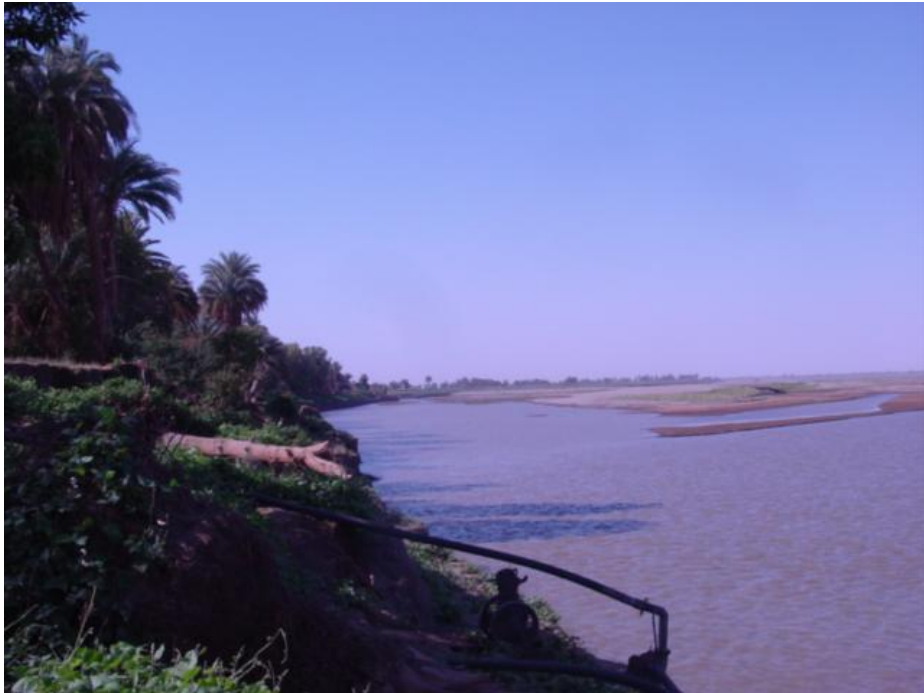
Figure 4- 12: River bank erosion along the Main Nile River (Barber area)
