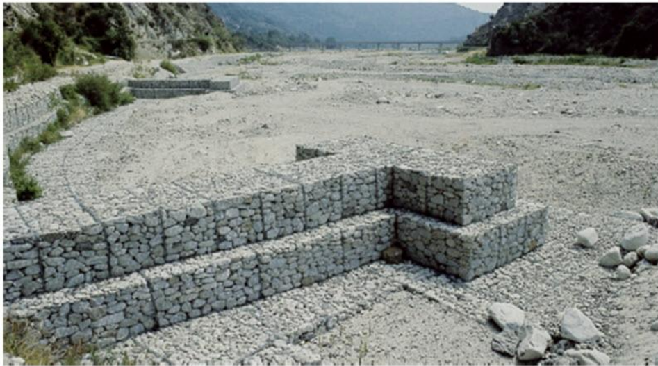
Figure 5-15: Typical gabion groynes in construction
