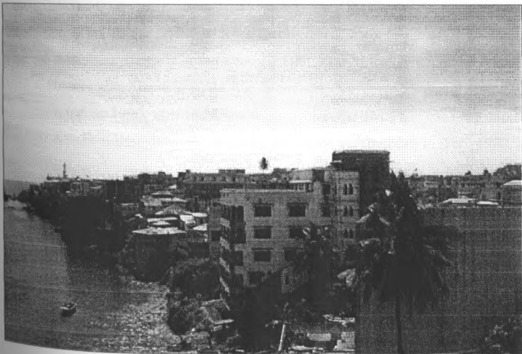
Views of the old town from the sea (source: http://archnet.org/library/ )
