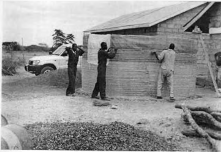
Maasai men building a water tank (skilled labour)
