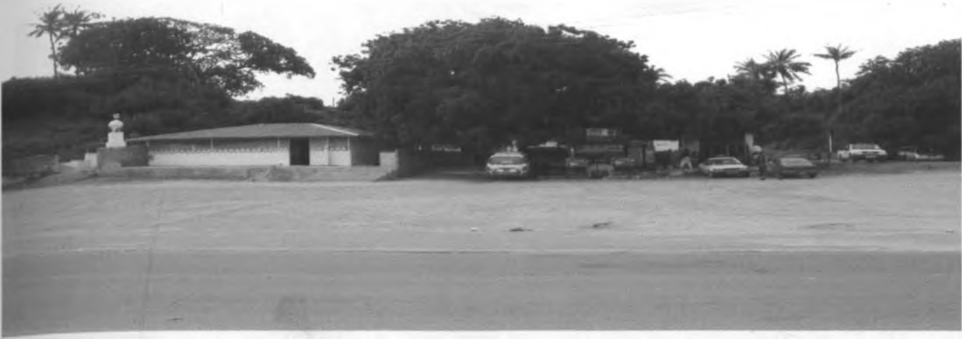
Plate 4.8.1, (b) Construction of a mosque within the site is a bad precedent.
