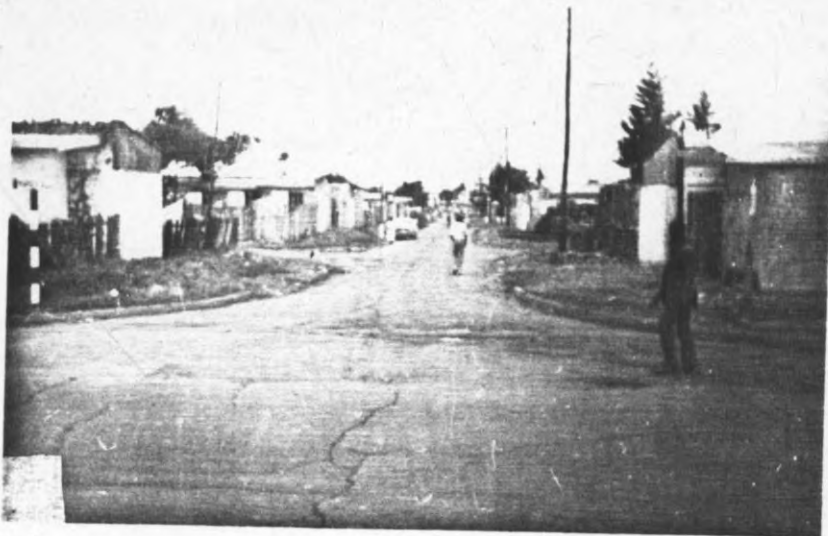
PLATE 9: A collector street in Umoja I Estate.
