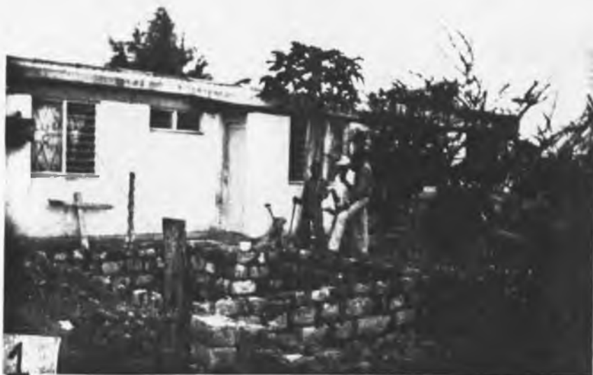
PLATE 1: Complete foundation for a front extension
