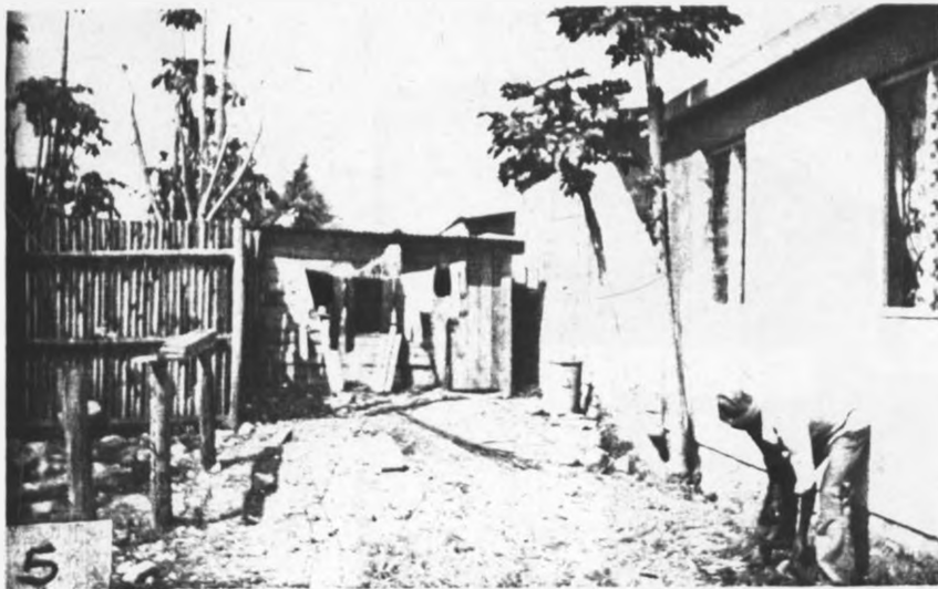
PLATE 5: A wooden back extension (Emphasise ineffectiveness of Development Control enforcement)
