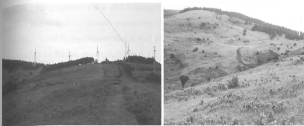
Photo 6.10: Ngong Hills and the Windmills used to generate Wind Energy
