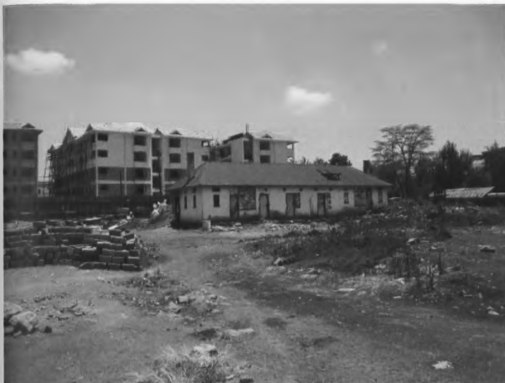
Plate 5.15: Ngara phase I and demolished old bungalow.
