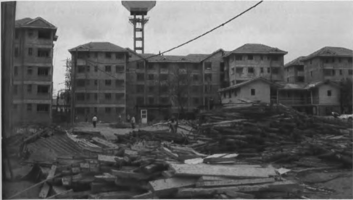
Plate 5.24: Ngara phase II with the raised water tank in the background.
