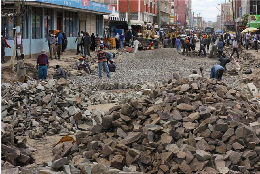
Figure 4.4.Rehabilitation of Second Avenue. Photograph by author
