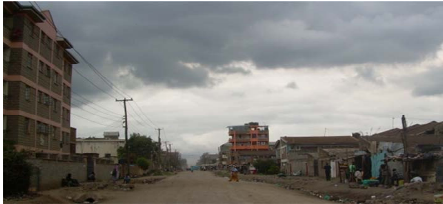
Figure 4.2. Rehabilitated General Waruingi street. Source: Photographed by author
