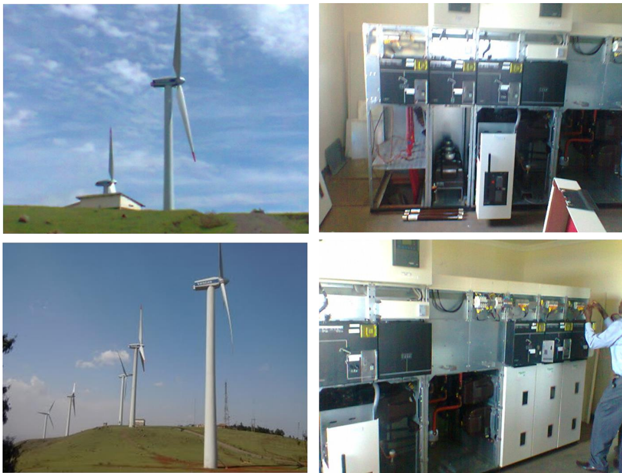
Figure 3.1 Maintenance work at the Ngong Wind Farm
