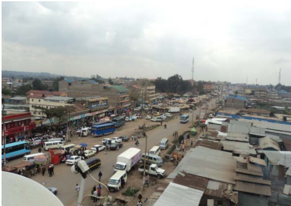
Plate 6-11: Magadi Road aerial view
