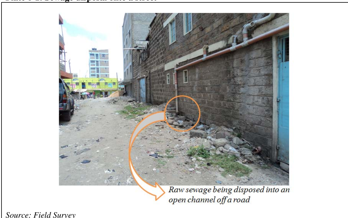
Plate 6-1: Sewage disposal onto a street
