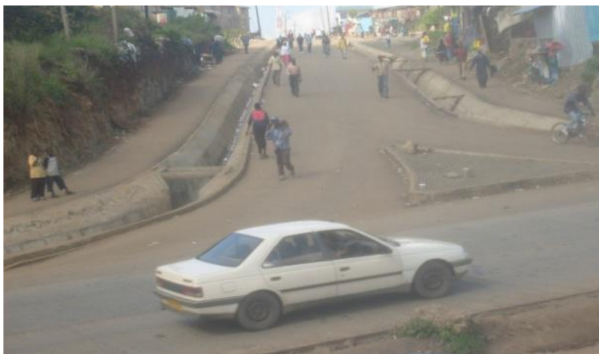
Figure 2: Access Road in Kibera Nairobi
