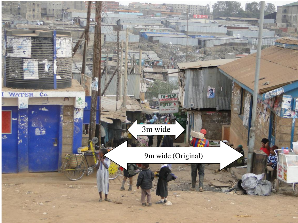
Figure 5.8 Encroachment on a Road Reserve
