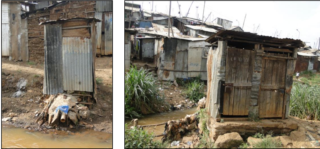
Plate 6: Toilet Facilities Serving the People Close to the River
