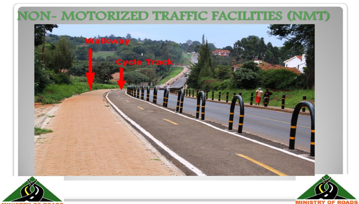
Figure 11: Non-motorized traffic facility
