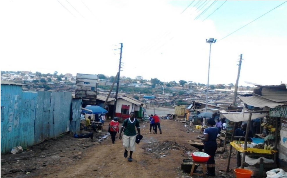
Figure 7: Poor infrastructure networks in Soweto East Village
