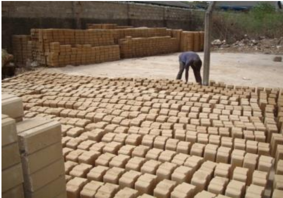
Stacking and curing of interlocking stabilized soil blocks.
