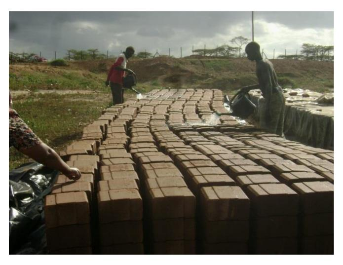
Plate10: Curing of ISSBs at the yard
