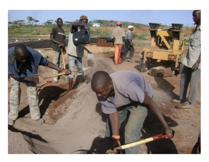
Plate7: Material Preparation for ISSBs production
