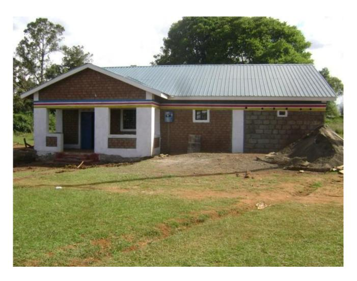
Plate11: ISSBs constructed police post
