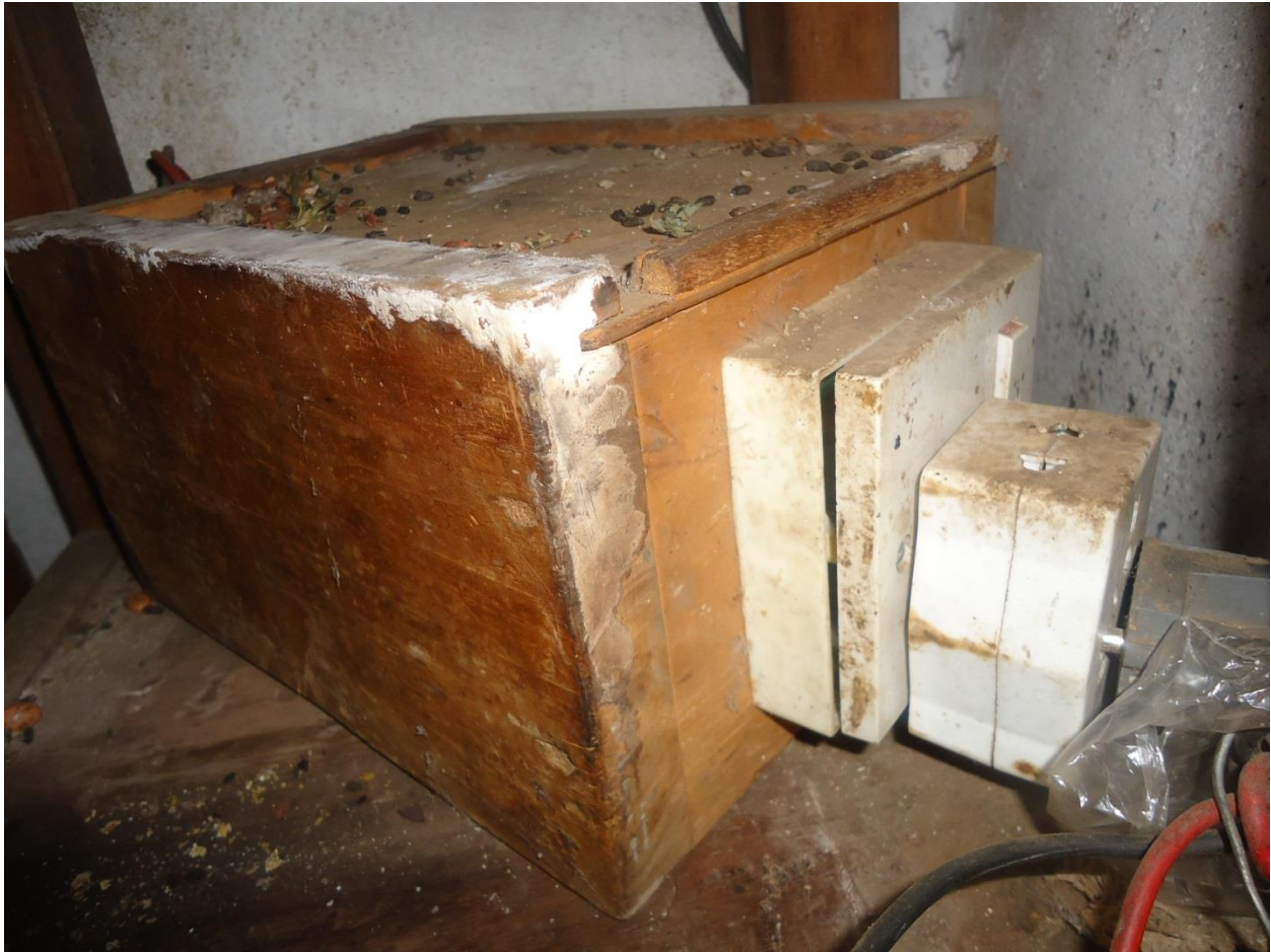
Figure 4.6: Solar Inverter in a Building
