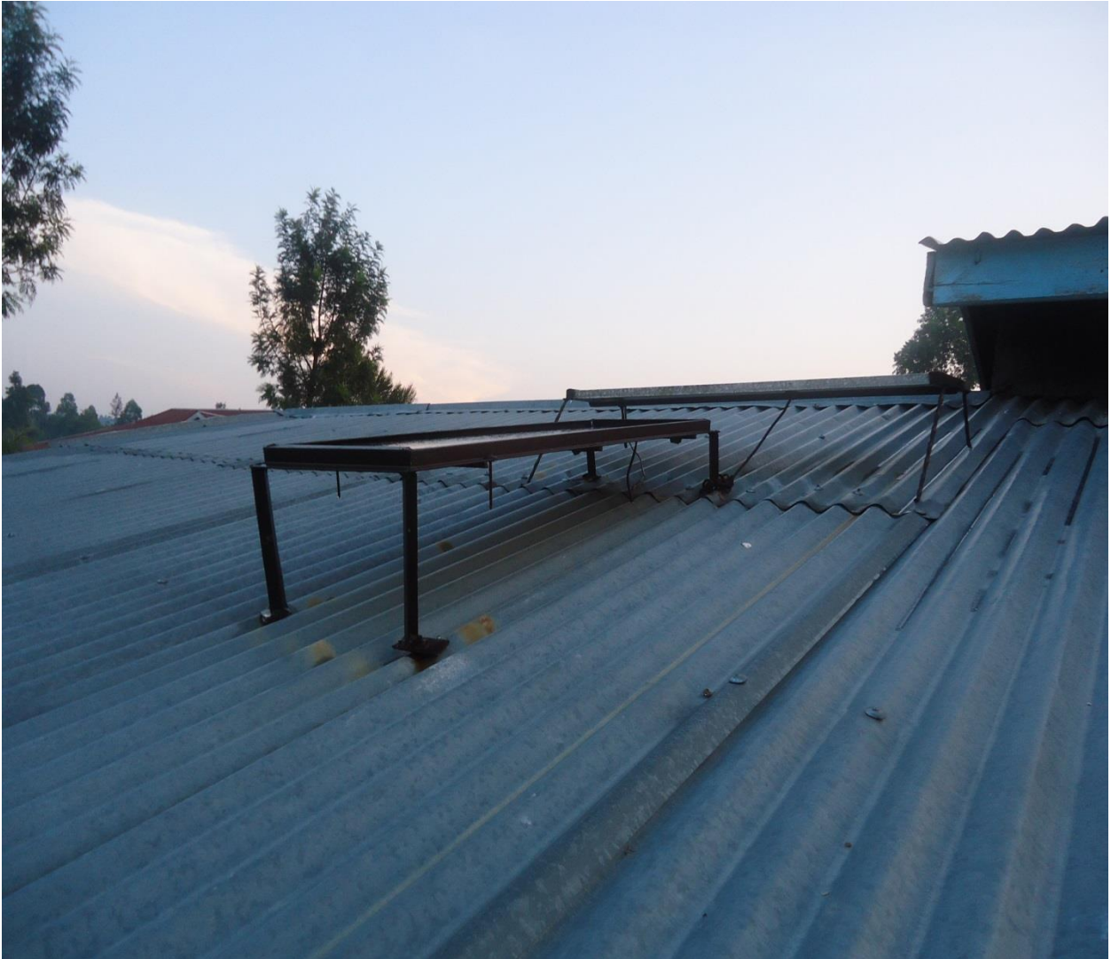
PV Solar installed on the roof using stands.
