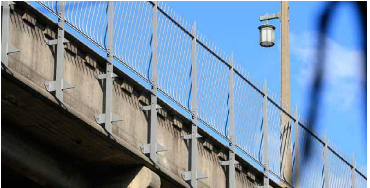
Picture 55: Bridge with sides protected by mesh
