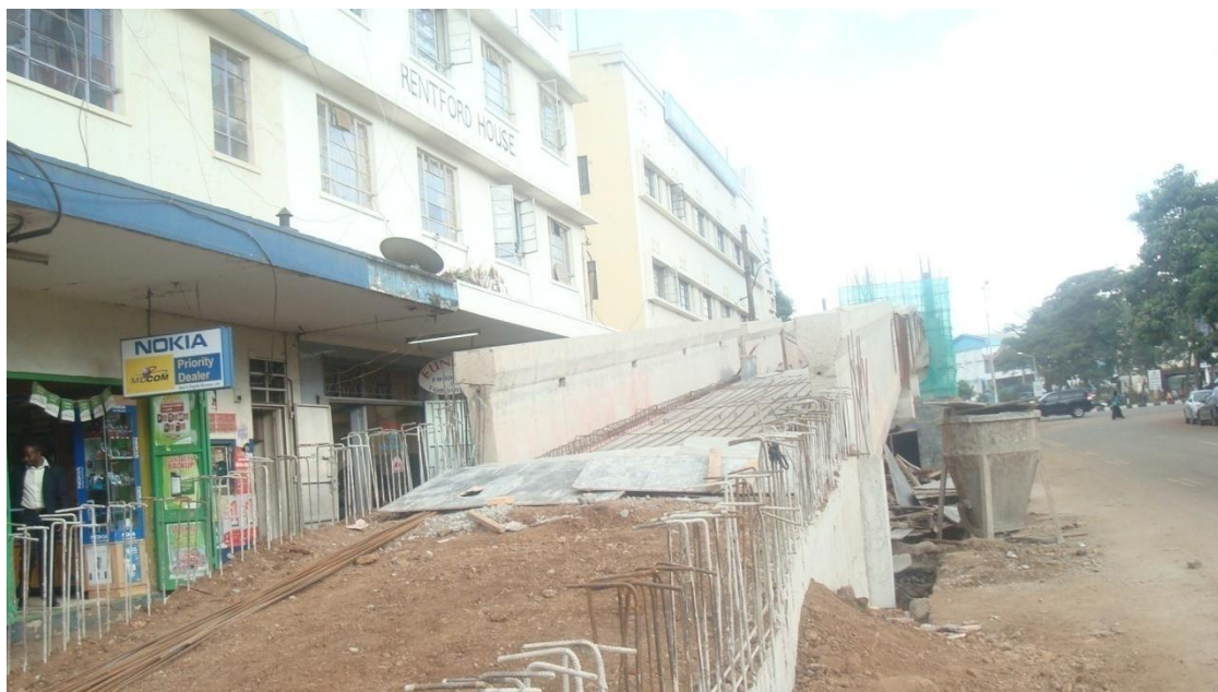
Picture 49: University of Nairobi PFB under construction
