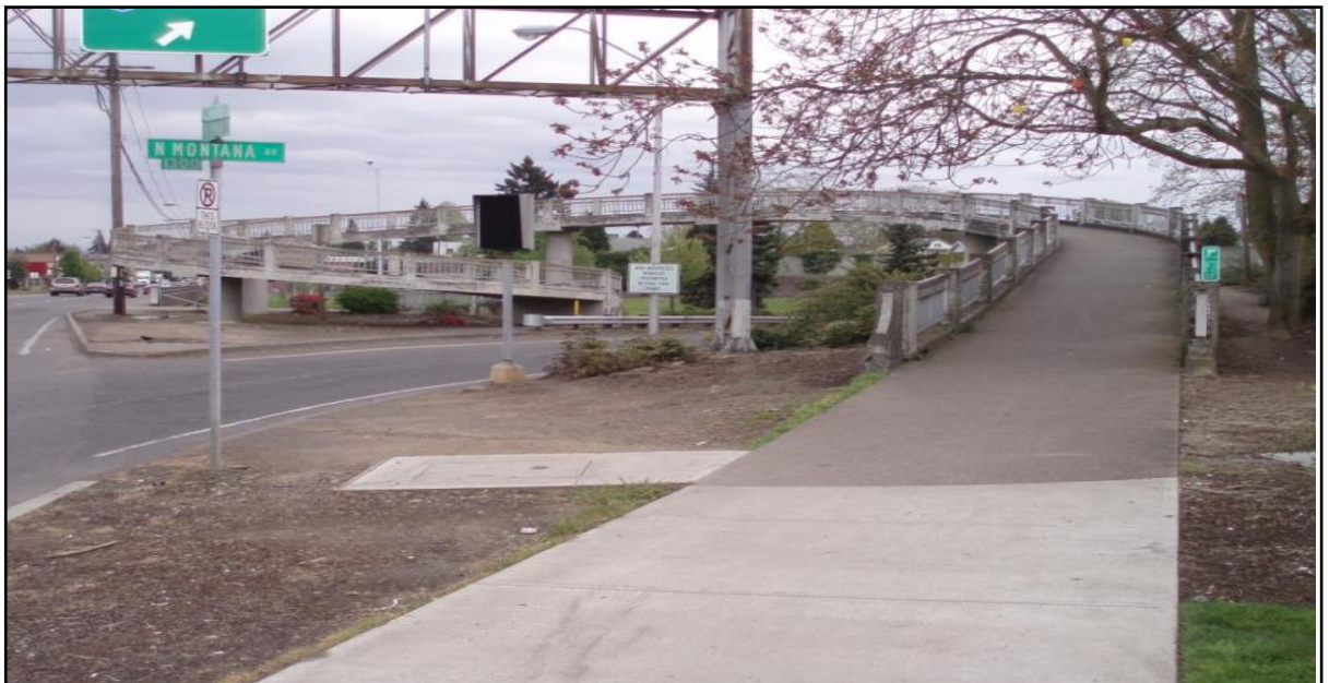
Picture 26: Pedestrian Overpass with ramp to cater for all users including the disabled
