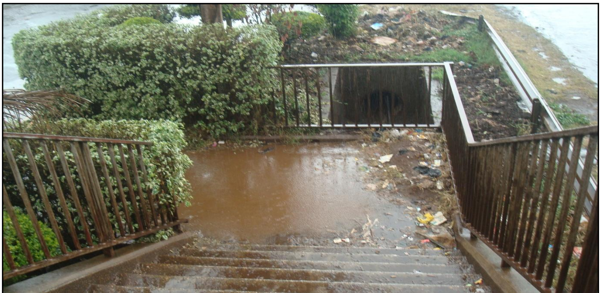
Picture 5: Southern end of Uthiru pedestrian footbridge with water
