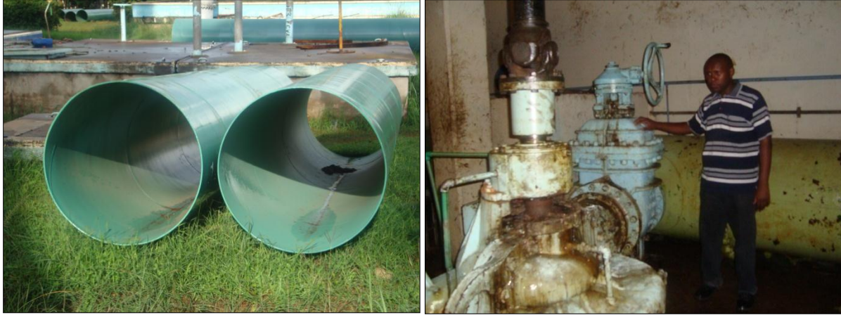
Fig 3-6: Steel pipes ready for lining and suction valve. Source (NCWSC)
