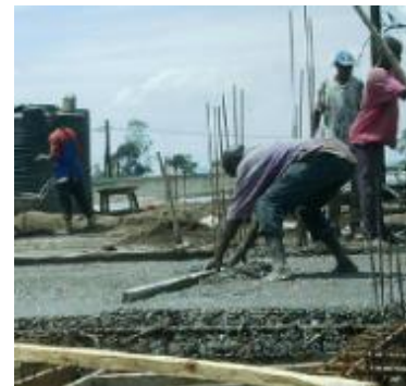
Figure 5: Finishing with straight edge, Siaya, 2010.
