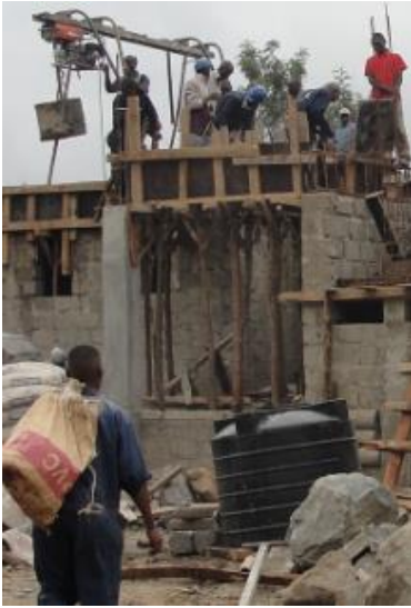
Figure 1: Hoisting concrete in a bucket, Nairobi, 2011.
