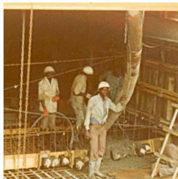
Figure 4: Placement by tremie and compaction by immersion vibrator, Mombasa, 1979.
