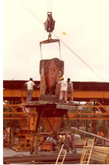
Figure 2: Hopper suspended from cable crane, Mombasa, 1979.
