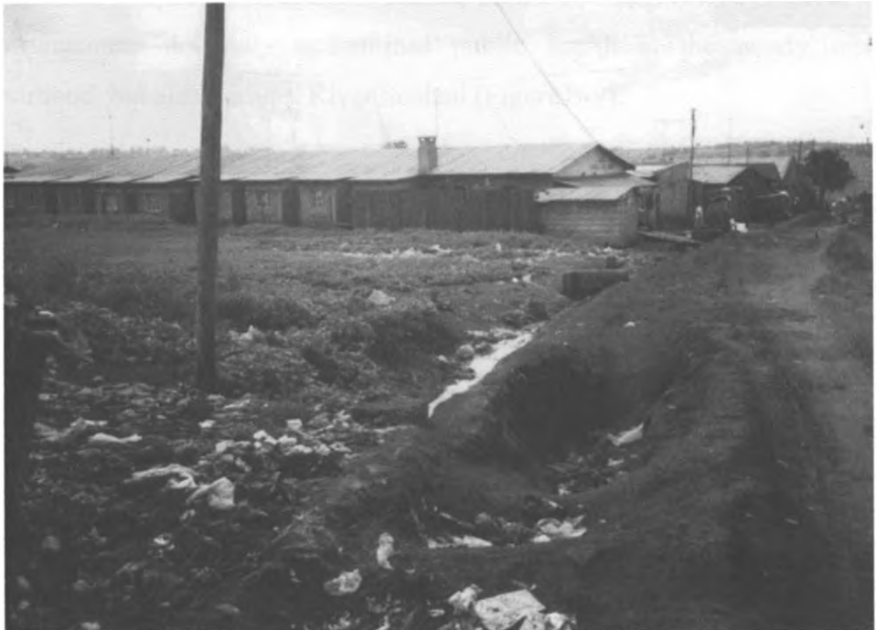
Plate 5-4: A Road in Poor Condition
