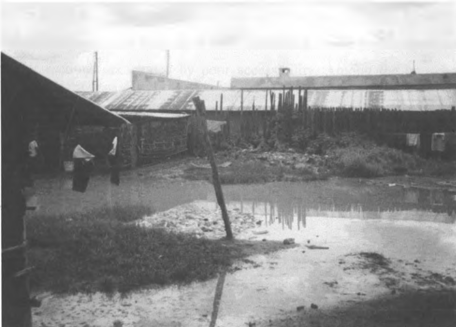
Plate 6-6: A Poorly Drained Compound
