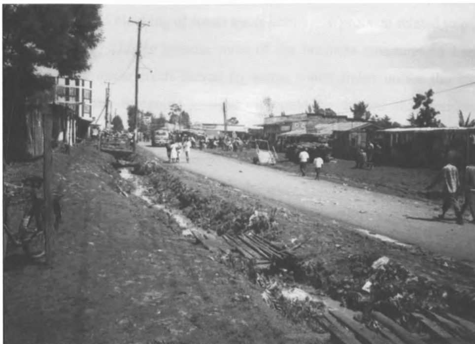
Plate 7-1: A Blocked Storm Water Drain
