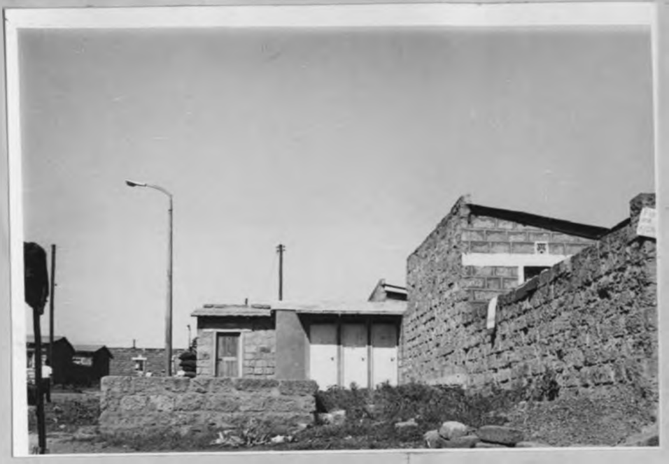
Plate No.5: The wetcore - kitchen, toilet and shower - provided to the builder allottee of type B plot.
