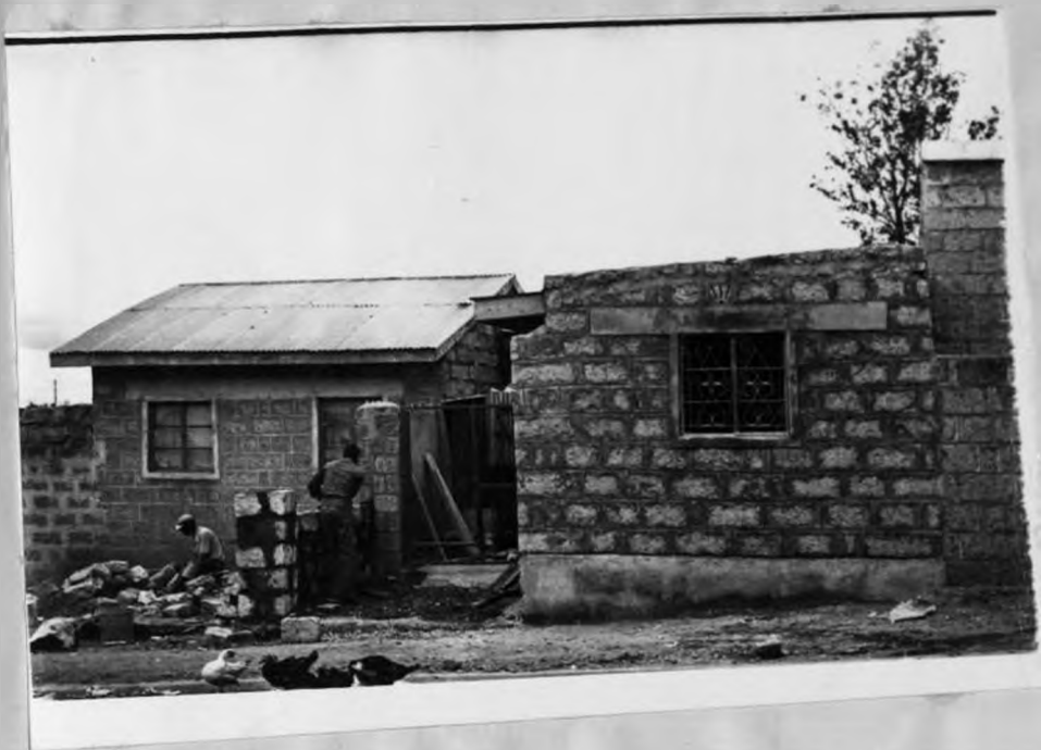
Plate No.7: Building construction continues in Dandora Phase one.
