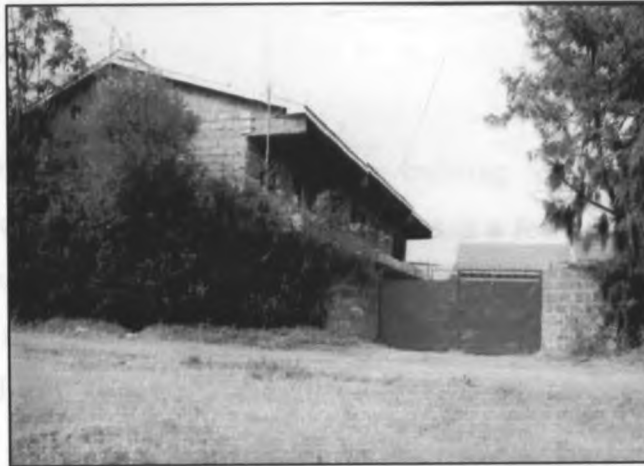
Plate 18 A residential compound with upcoming flats
