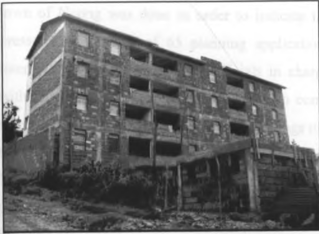
Plate 17 Contravention of rear setbacks. The stone wall marks plot boundary
