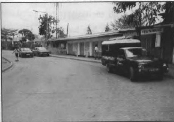
Plate 19 Construction on Road Reserves
