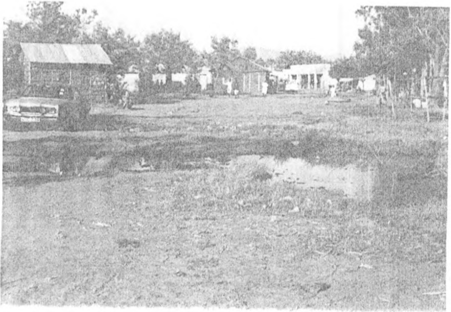
Plate 8: Buildings requiring structural improvement in the background and waterlogged road in the foreground (part B)
