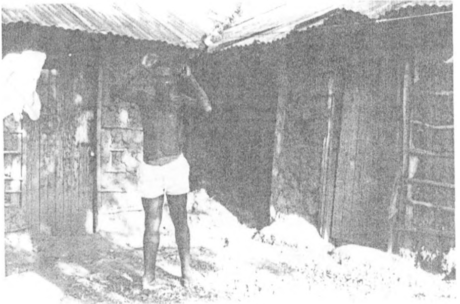
Plate 4 A dilapidated building in part B
