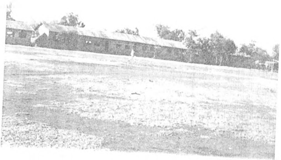
Plate 15: Poorly maintained Mauvatta primary school in part A
