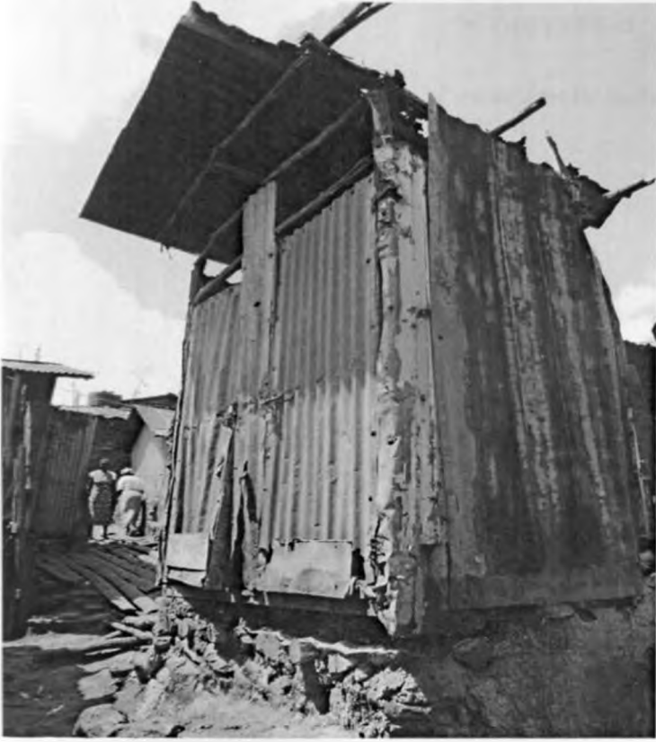
A shared toilet in one of the plots in Kibera
