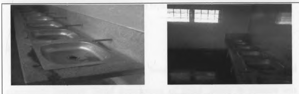
Toilets and washrooms
