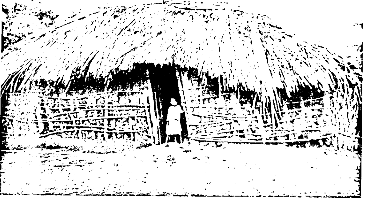
Figure 2.3 Stick and mud built house in Taveta, Tana River and Kwale districts
