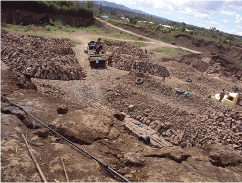
Figure 1. Rough ashlars being loaded onto trucks in one of the stone quarries of Nairobi to be carted to building sites.
