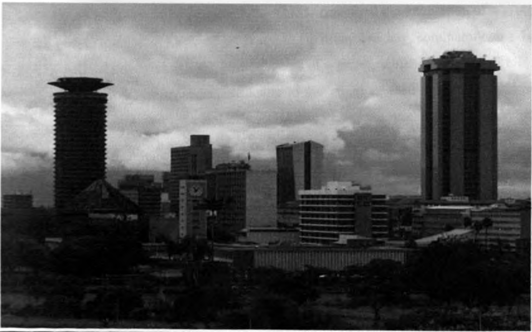
Plate 1.1: View of unique buildings near the Aga Khan Walk
