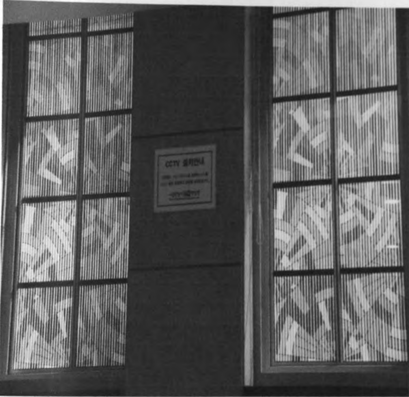
Figure 5.2: Picture of DSSCs used to make energy-generating windows in Korea.
