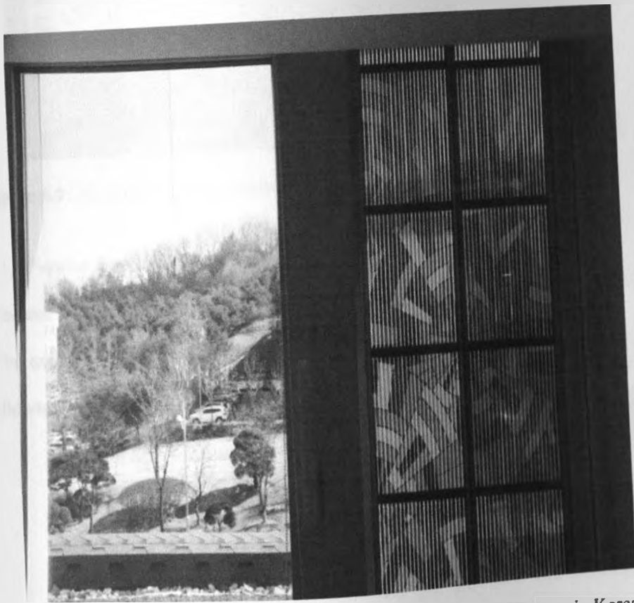
Figure 5.1: Picture of DSSCs used to make an energy-generating door in Korea.
