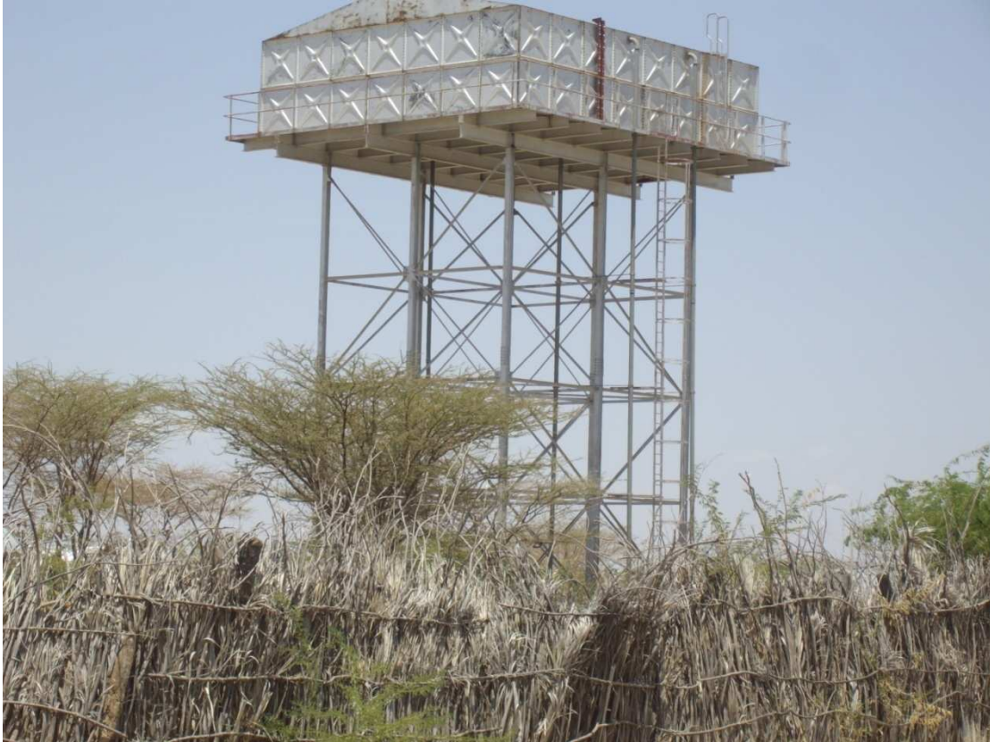
Plate 18: Water storage and supply tank
