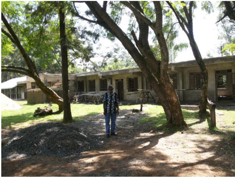
Plat E 5: Ongoing project Lab /Tuition Ingotse high school Navakholo Constituency
