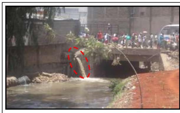
Plate 2.3: Direct Discharge of Sewer into the Nairobi River
