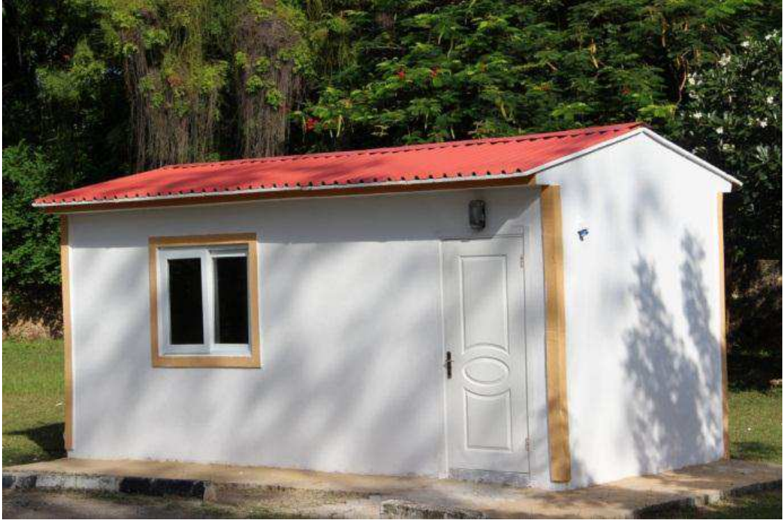
Figure 4.1: A bedsitter located within Elsek & Elsek office compound in Links road, Nyali – Mombasa
