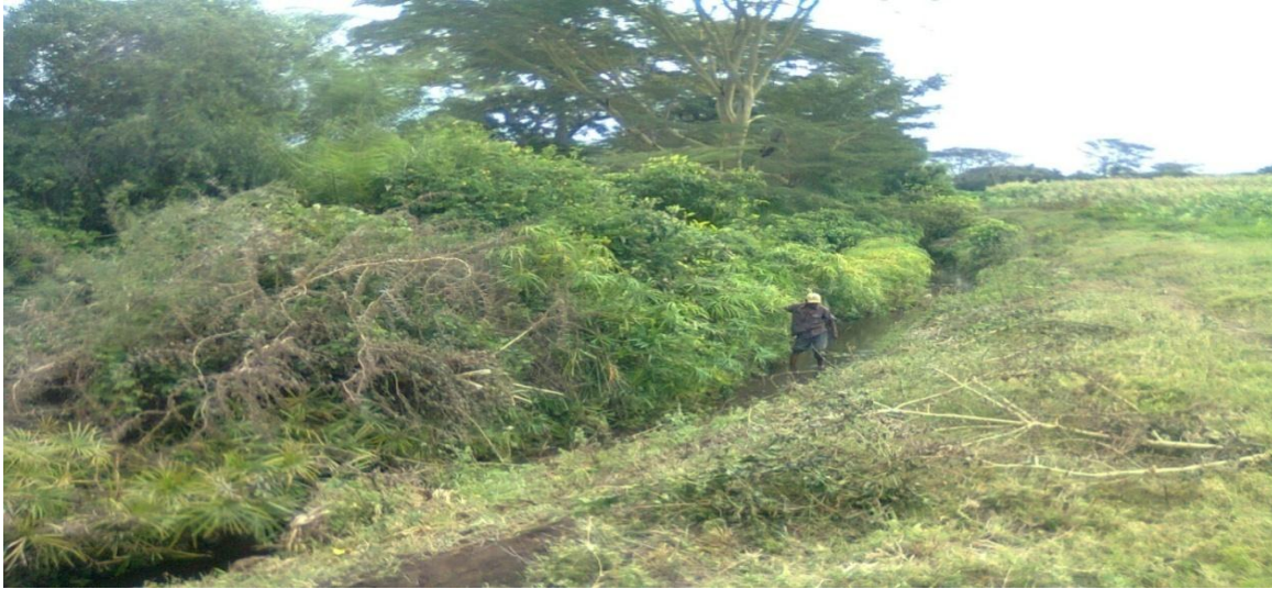
Plate 6: Clearing aquatic vegetation from irrigation canals
