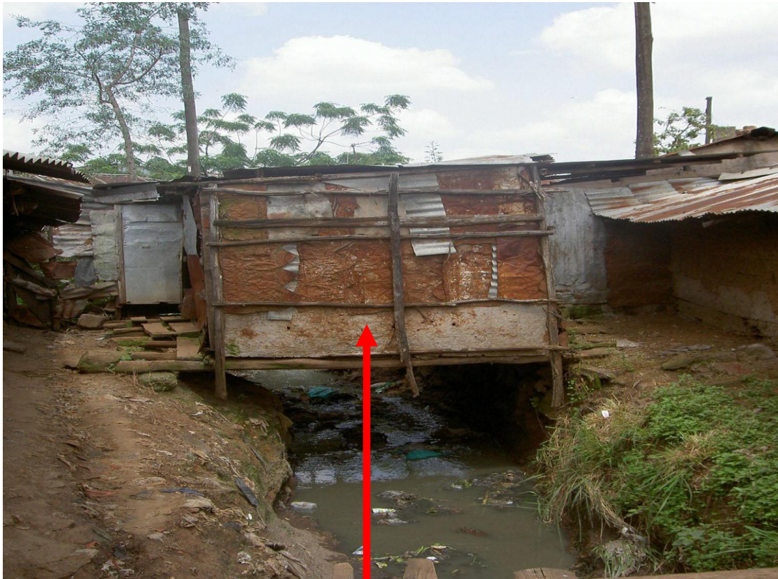
A Pit latrine constructed across a river channel
