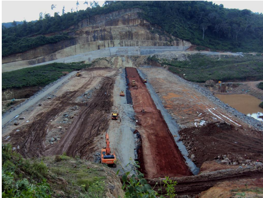
Plate 2-5: Chemususu Dam under Construction
