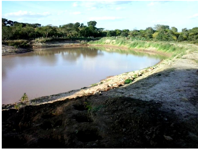
Plate 2-2: Kwa Ngii Dam Embankment
