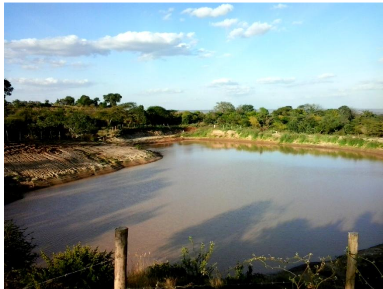
Plate 2-1: Kwa Ngii Dam Reservoir
