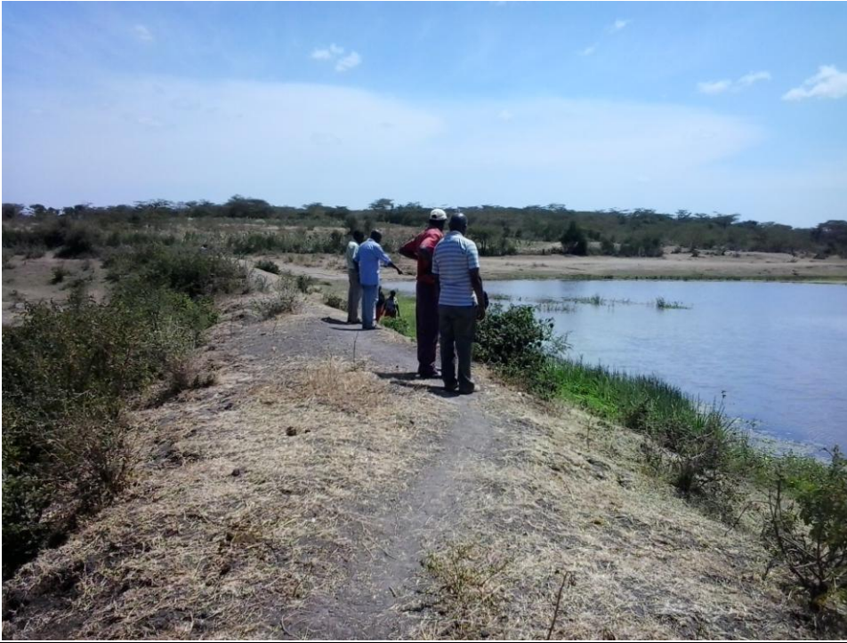
Plate 4-3: Typical Dam Embankment in the Research area
