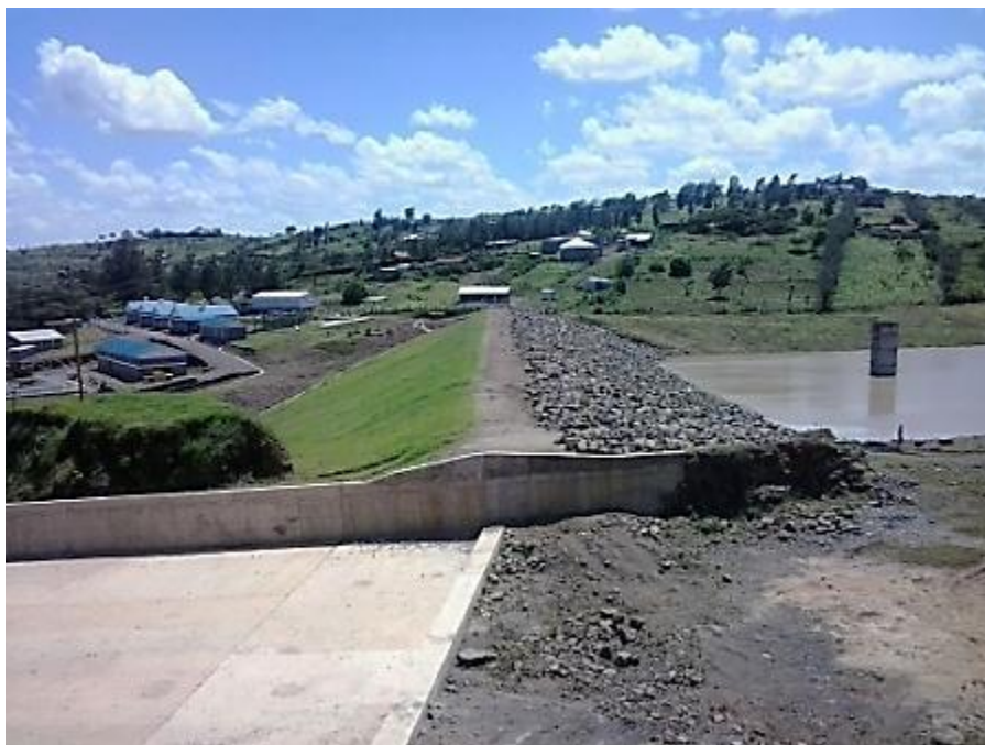
Plate 2-3: Kiserian Dam in Kajiado, Kenya
