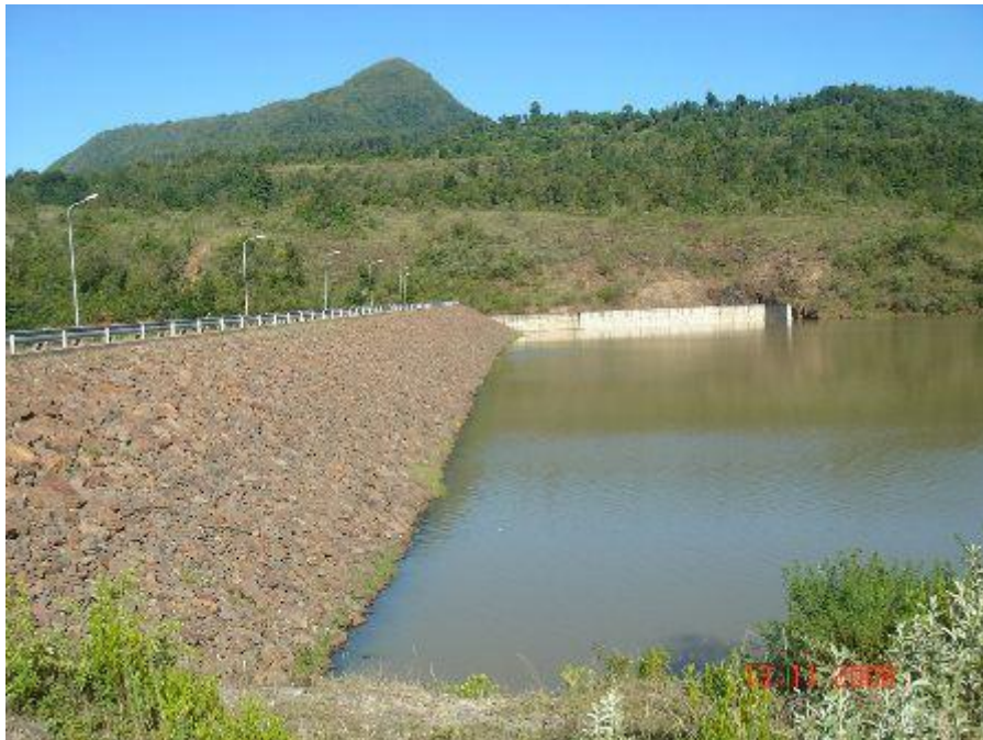
Plate 2-4: Kirandich dam, Kenya
