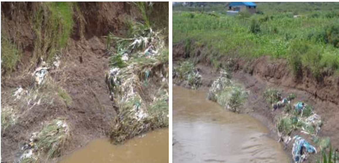
Plate 4.2 i: Basal Cleanout of the inner bank. Plate 4.2 j: Basal Cleanout of the outer bank Source: Researcher, (2013)
