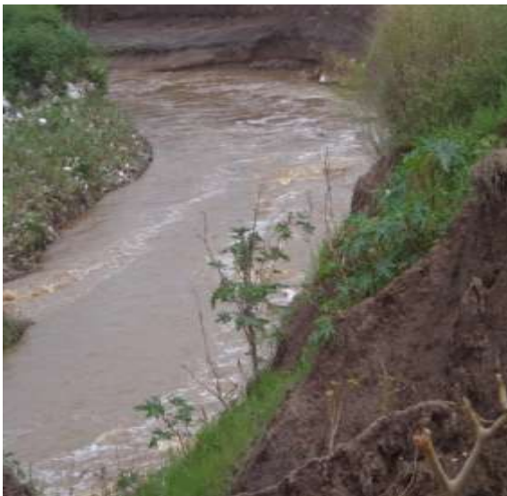
Plate 4.2 e: Undercutting of outer bank
