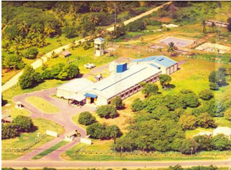
Figure 4-1: The MFPL Plant
