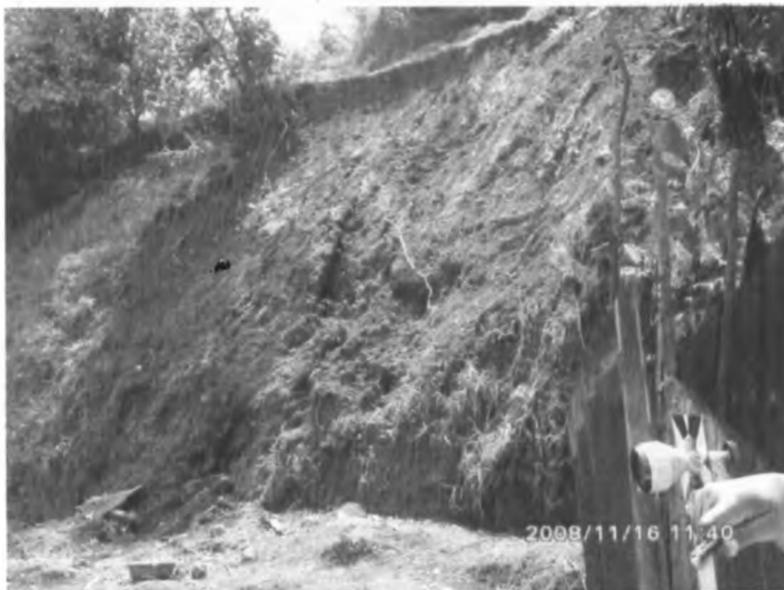
Figure 3.6: Right Side View of Mung'aria Village Landslide
