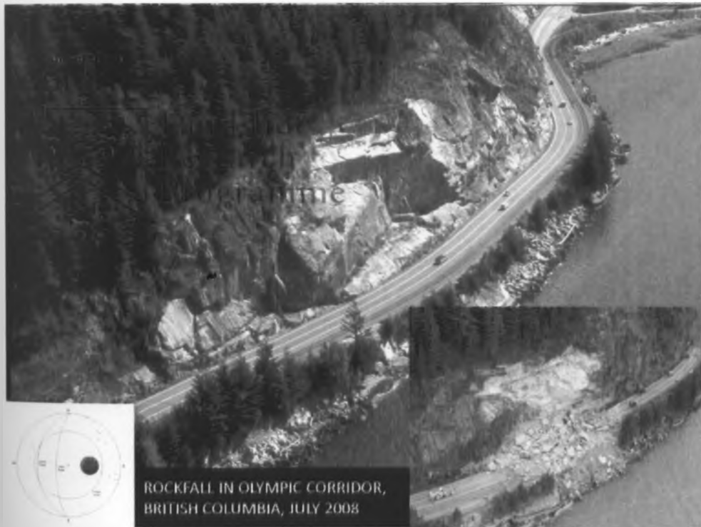
Fig. 2.24: Image showing the exact location of the failed cliff in 1997 and the subsequent failure in July, 2008 (LRP, 2008; inset Canadian Press, 2008)
