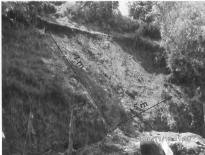
Figure 3.5: Left Side View of Mung'aria Village Landslide
