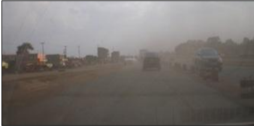
Plate 1: Section of the road on Lot 3 with a lot of dust posing health problems to the motorists and neighboring communities
