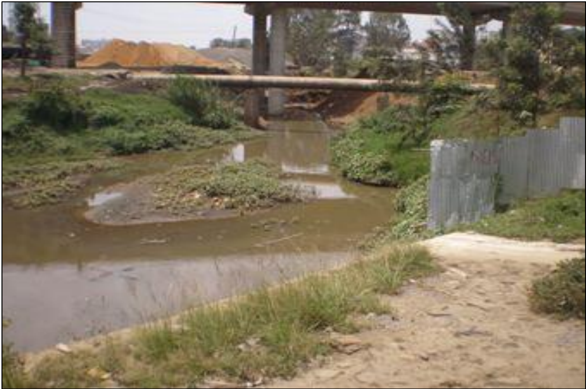
Plate 19: A Severely degraded Nairobi River channel due to dumping of waste into the river
