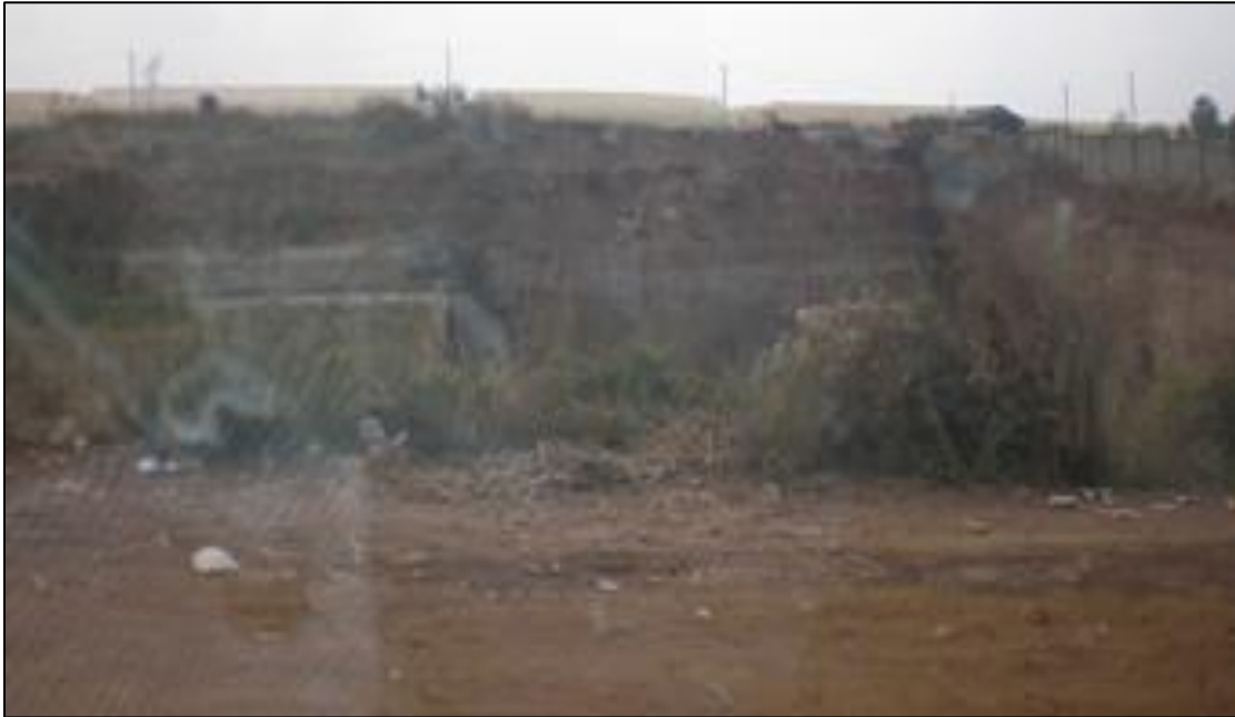
Plate 9: Open quarries and excavations posing health hazards to passer-bys in the area
