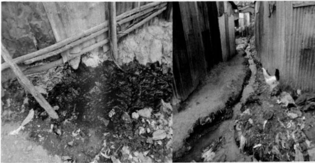
Plate 4.3 Poor drainage in the slum areas
