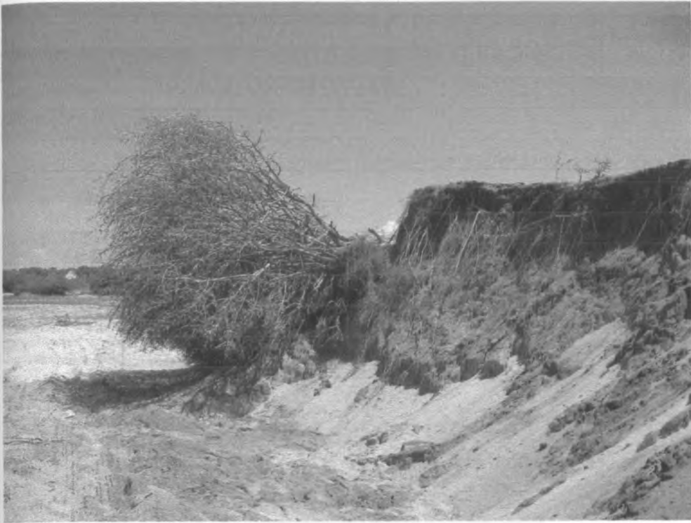
Plate 5: Loss of vegetation through edge effect in the mined areas
