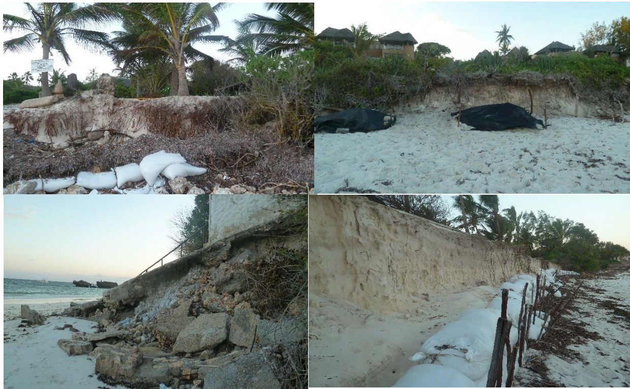
Figure 11 : Adjacent properties affected by erosion displaced by sea walls and other fortifications
