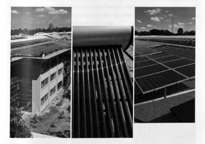
Plate 2.1: the Roof of the Entire Building covered by 1600m<sup>2</sup> of Photovoltaic Panels and Solar Water Heating Equipment
