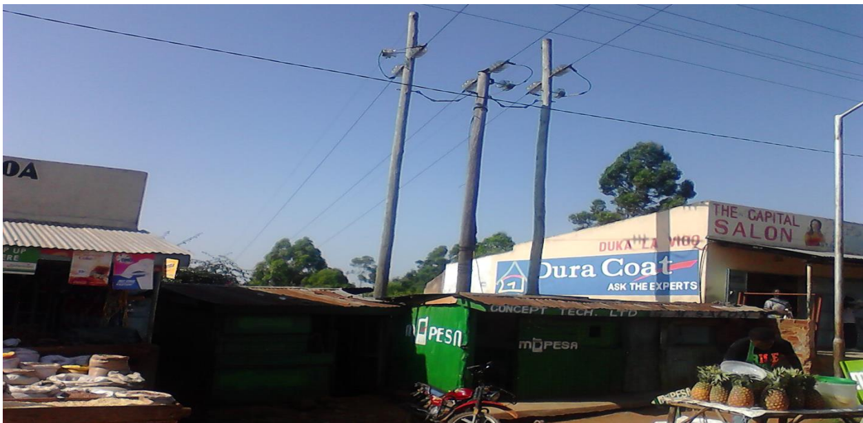
Plate 4.9: Buildings Under High Voltage Power Lines
