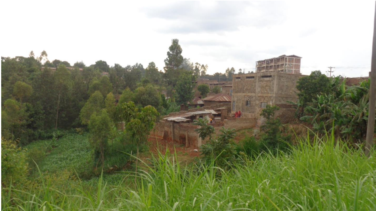
Plate 4.8: Commercial Building on a Planned Cemetery
