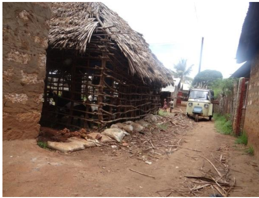
Use of filled bags to minimize the effect of flooding.
