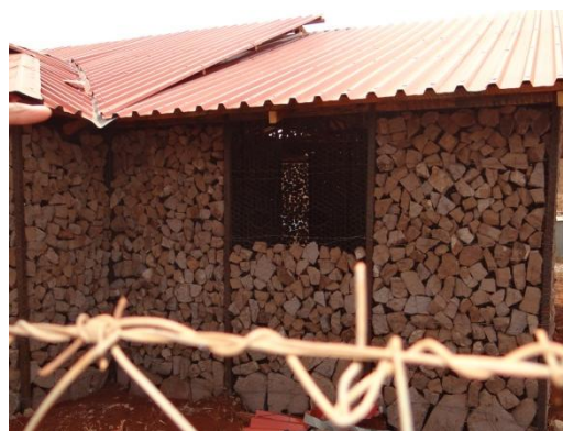
Stones and birbed wire technique as used in building.
