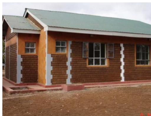
Building made of the stabilised interlocking blocks
