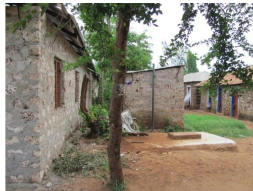
Minute septic tanks in parts of Muyeye.
