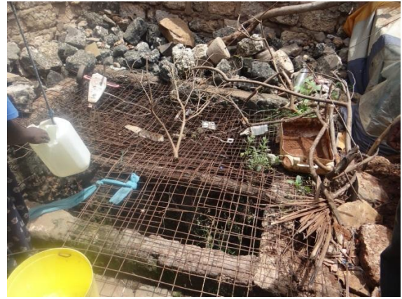
Unsafe water supply
