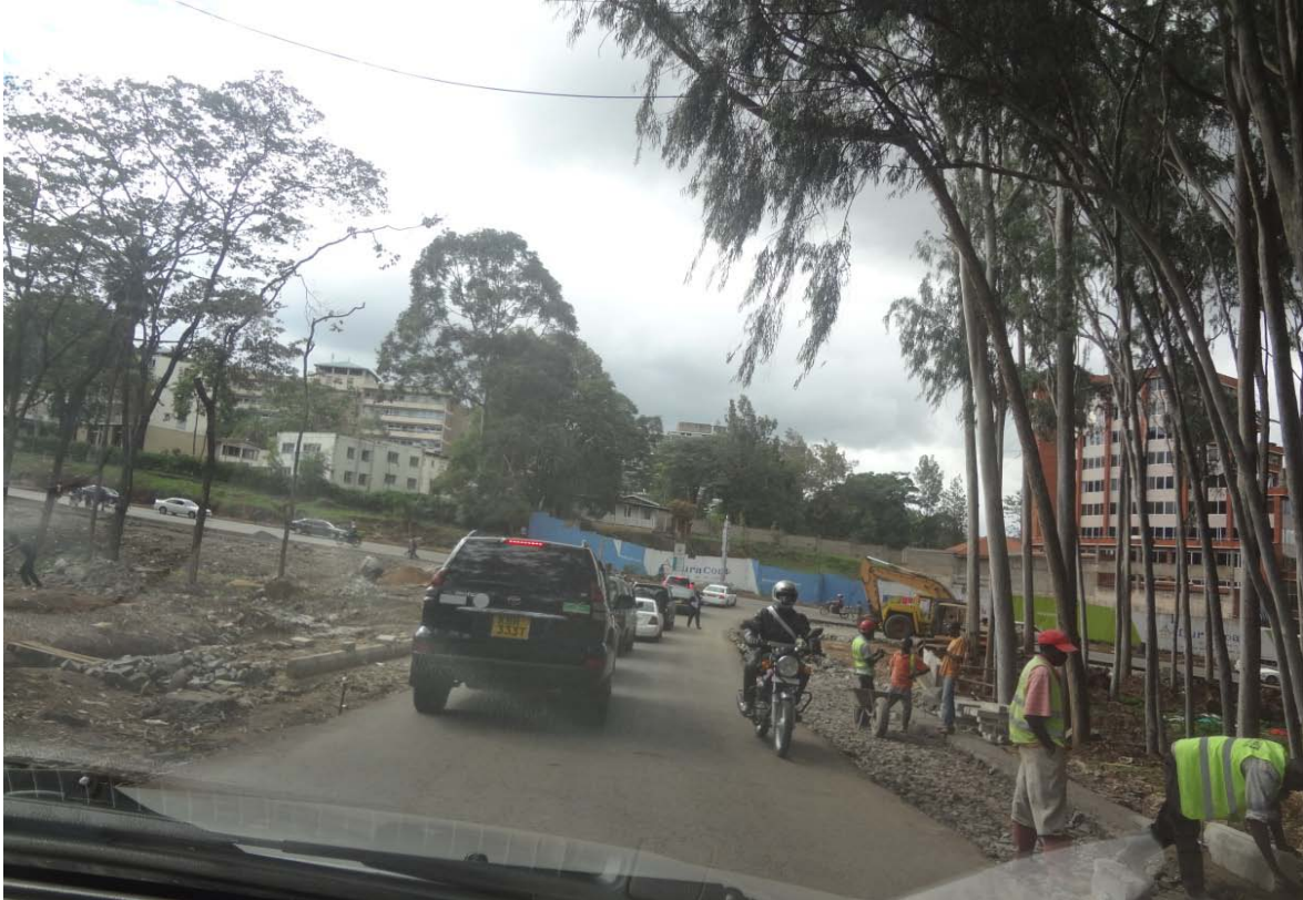
Figure 2.2: Road widening at Lower Hill and Haille Selassie Avenue junction
