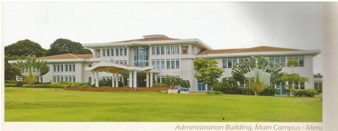
Administration block, opened on 10.9.2002.
